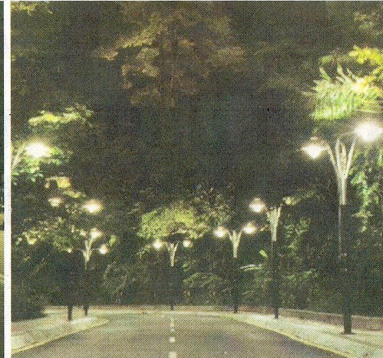
■ Correct choice of lamp posts. ■ The light on both the walkways and the street is not blocked by trees. ■ No dark shadows on the street, instead the street is well-lit.
